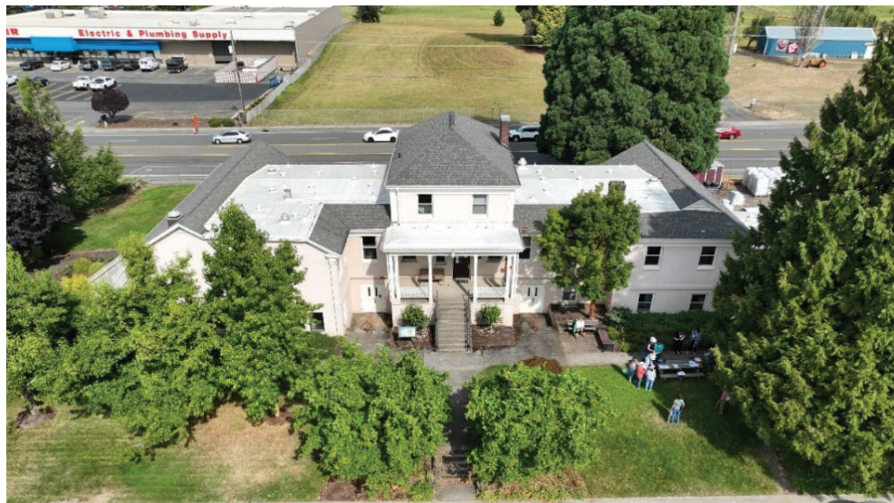
78 th Street Heritage Farm Administration Building
