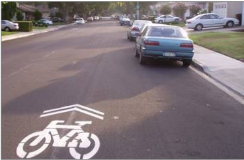
Figure 8. Shared lane markings are used to indicate a bicycle route, and to show cyclists where they should be riding in the road.
