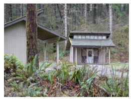
Figures 6 & 7. The old camping shelters have been repaired, repainted and enclosed to help reduce weathering damage.
