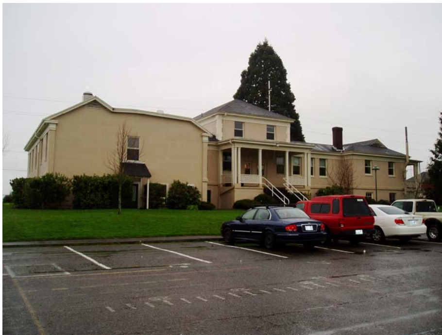
Figure 10. View of the Clark County Poor Farm Main Building, south (rear) elevation. The view is to the north-northeast.
