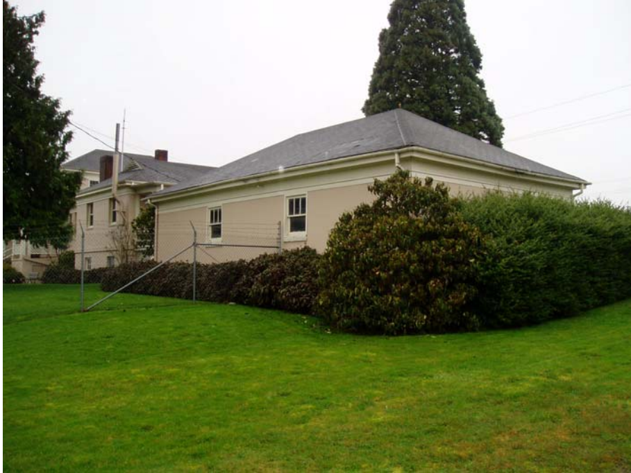
Figure 17. Detached garage, built 1926. South (left) and east (right) elevations, view to the northwest.
