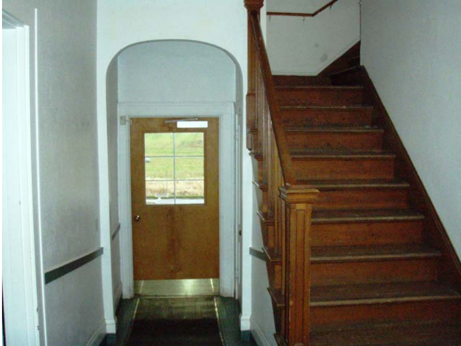
Figure 12. Interior view of central entry hall, reverse view from Figure 11, facing south.
