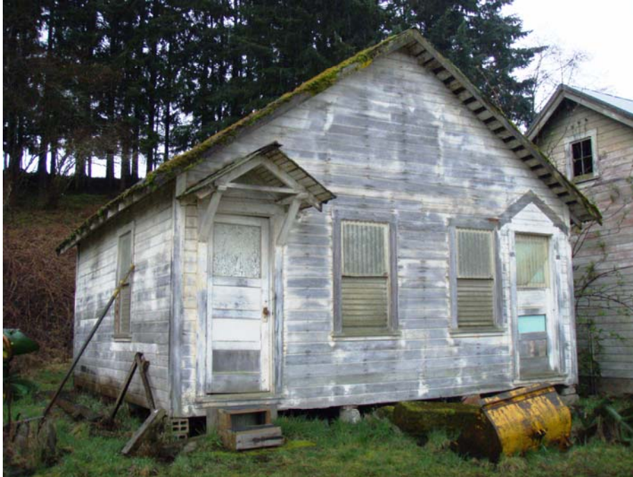
Figure 21. Bunk House, east (left) and north (right) elevations. The view is to the south-southeast.
