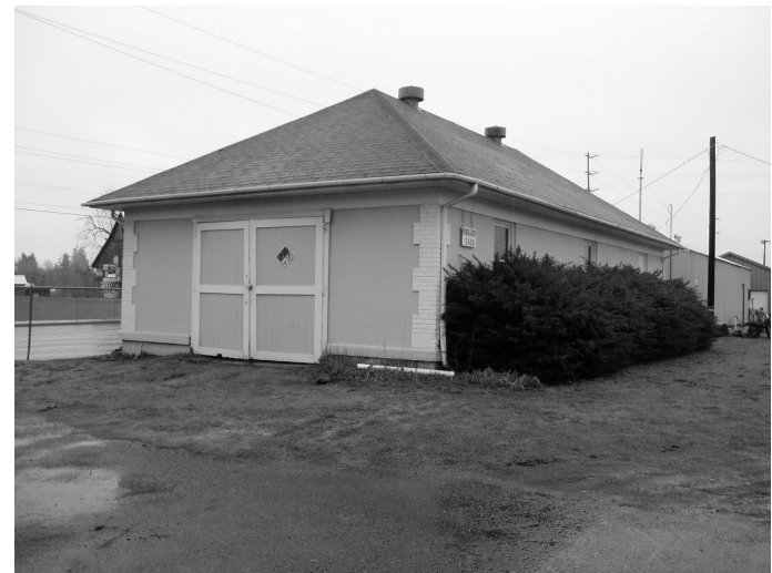
View of Clark County Poor farm Milk House, view to the northeast taken 2/26/2010
