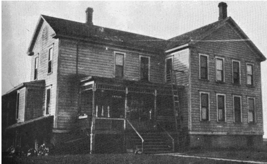
Figure 3. Ca. 1895 Poor Farm building, east side, view to the northwest.
