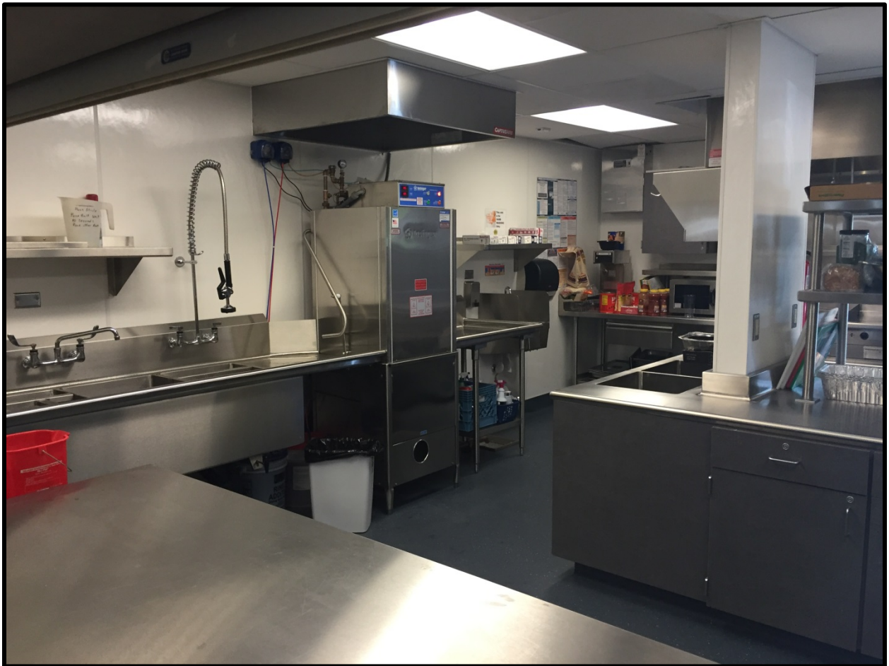
Washougal Community Center Kitchen Remodel
