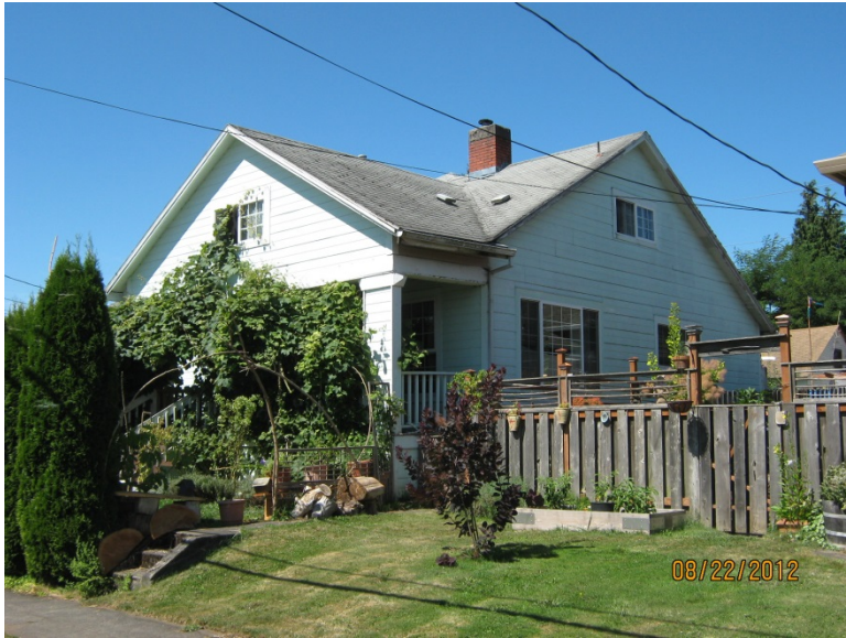
Housing Rehabilitation Before
