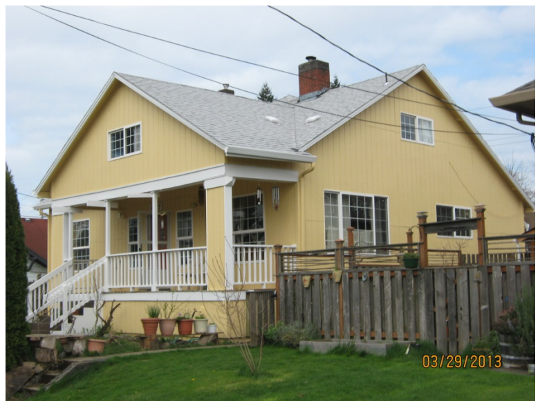
Housing Rehabilitation After
