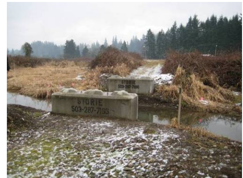
Location of culvert removal on Manley Creek.
