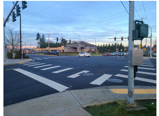
Highway 99 Pavement Improvements (NE 78th Street - NE 134th Street)
