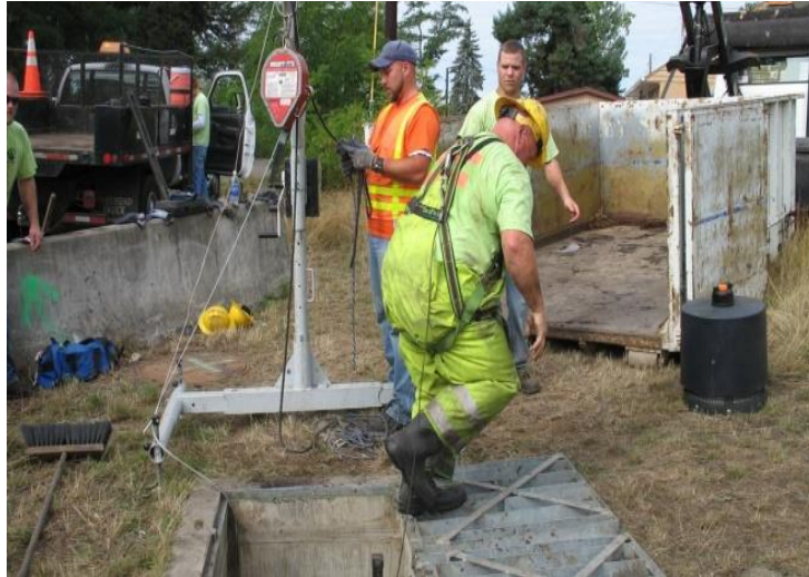
County crew replacing filters in a stormwater filter vault system
