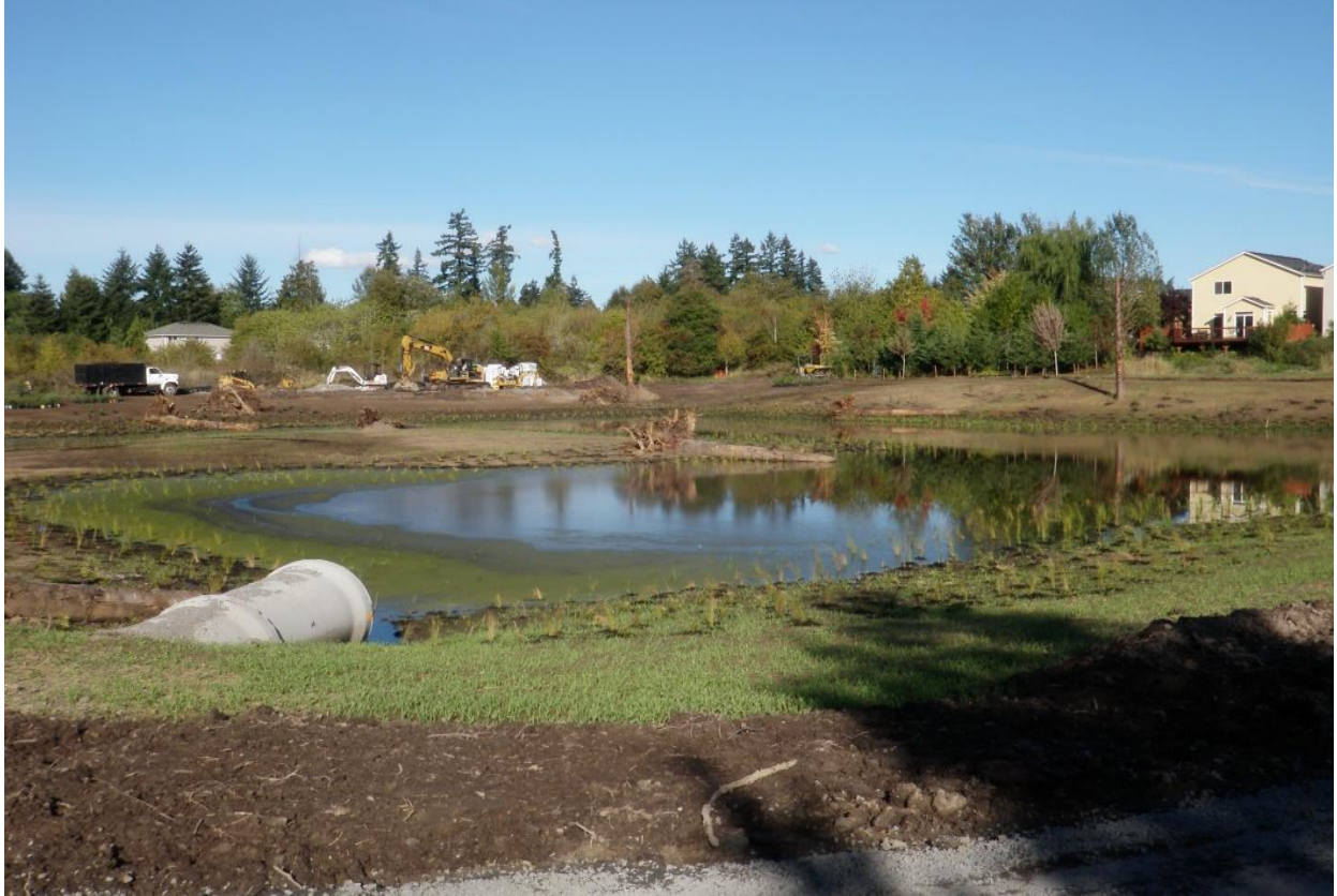
Construction of the Thomas Wetland East Stormwater Facility
