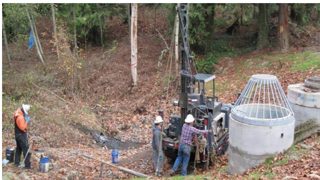
Encore Stormwater Facility Retrofit
