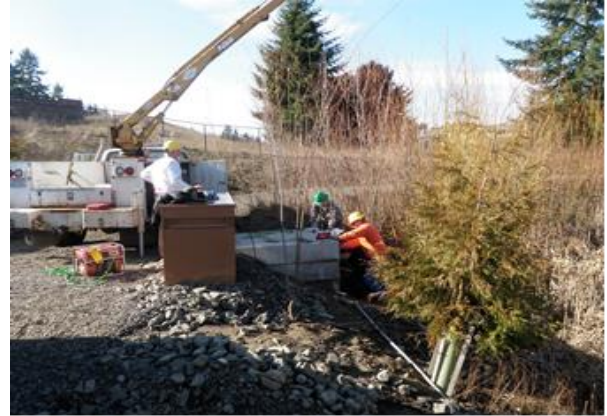
Crews install weir at a treatment wetland BMP monitoring site
