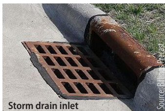
Storm drain inlet
