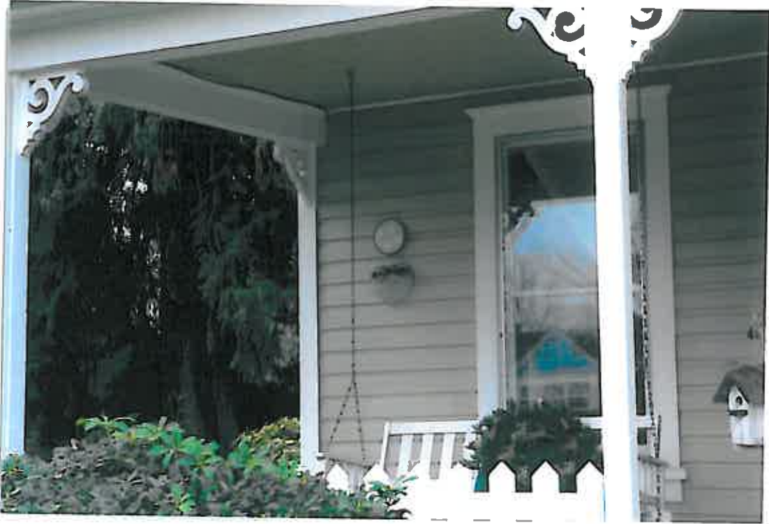
Covered front porch North side
