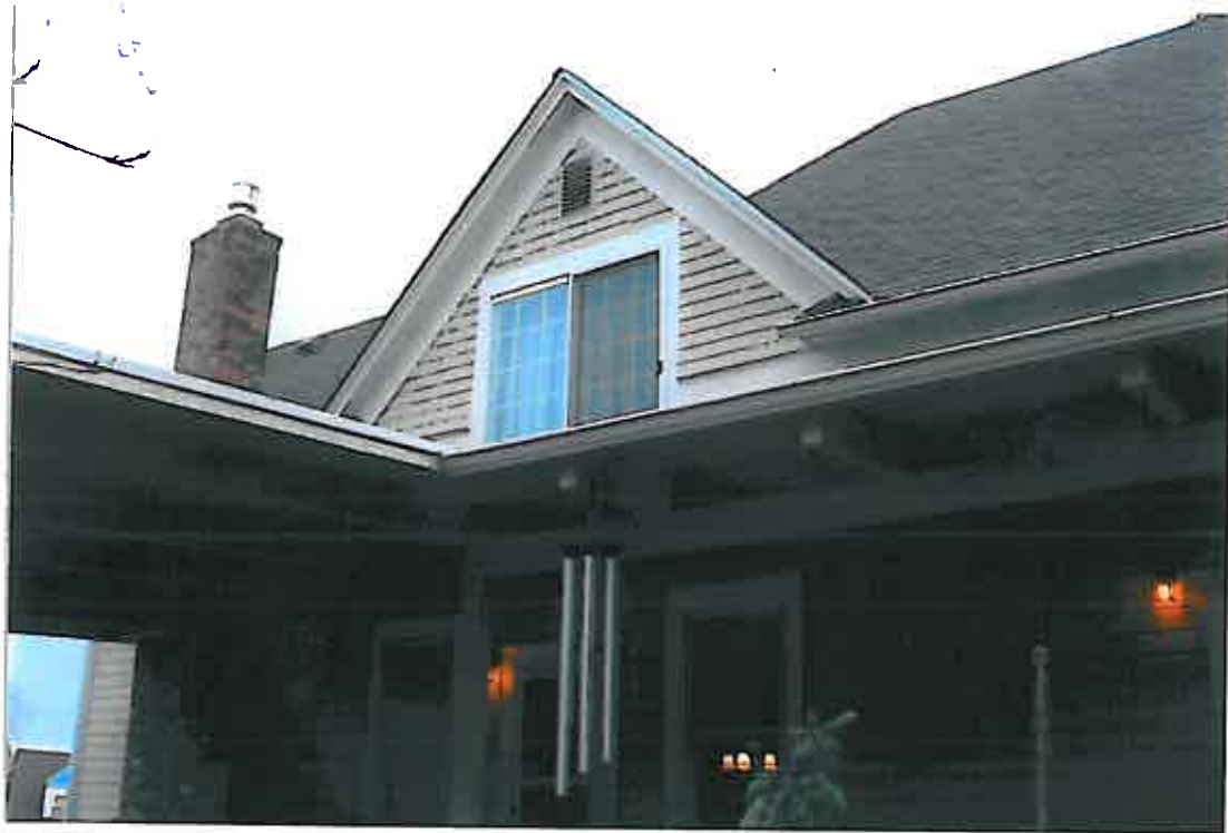
Looking at West side 2nd Story
