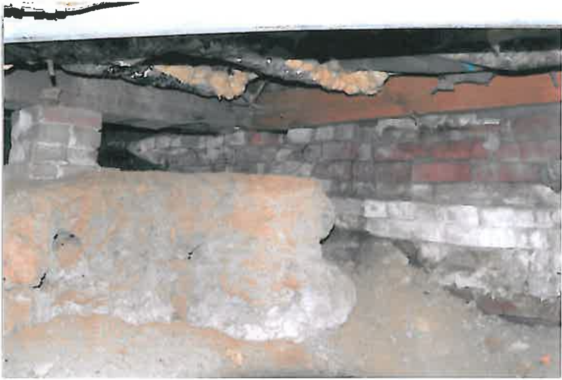
Brick Foundation (Top) South side
