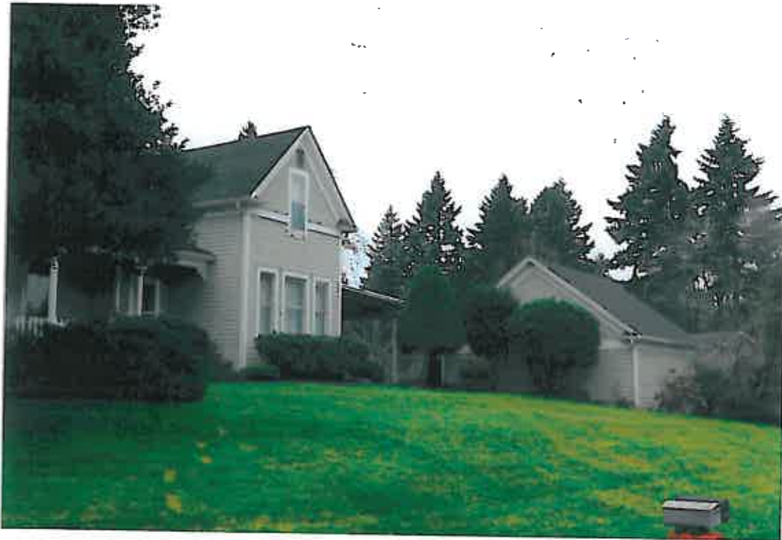
Looking at front and garage from Northeast corner
