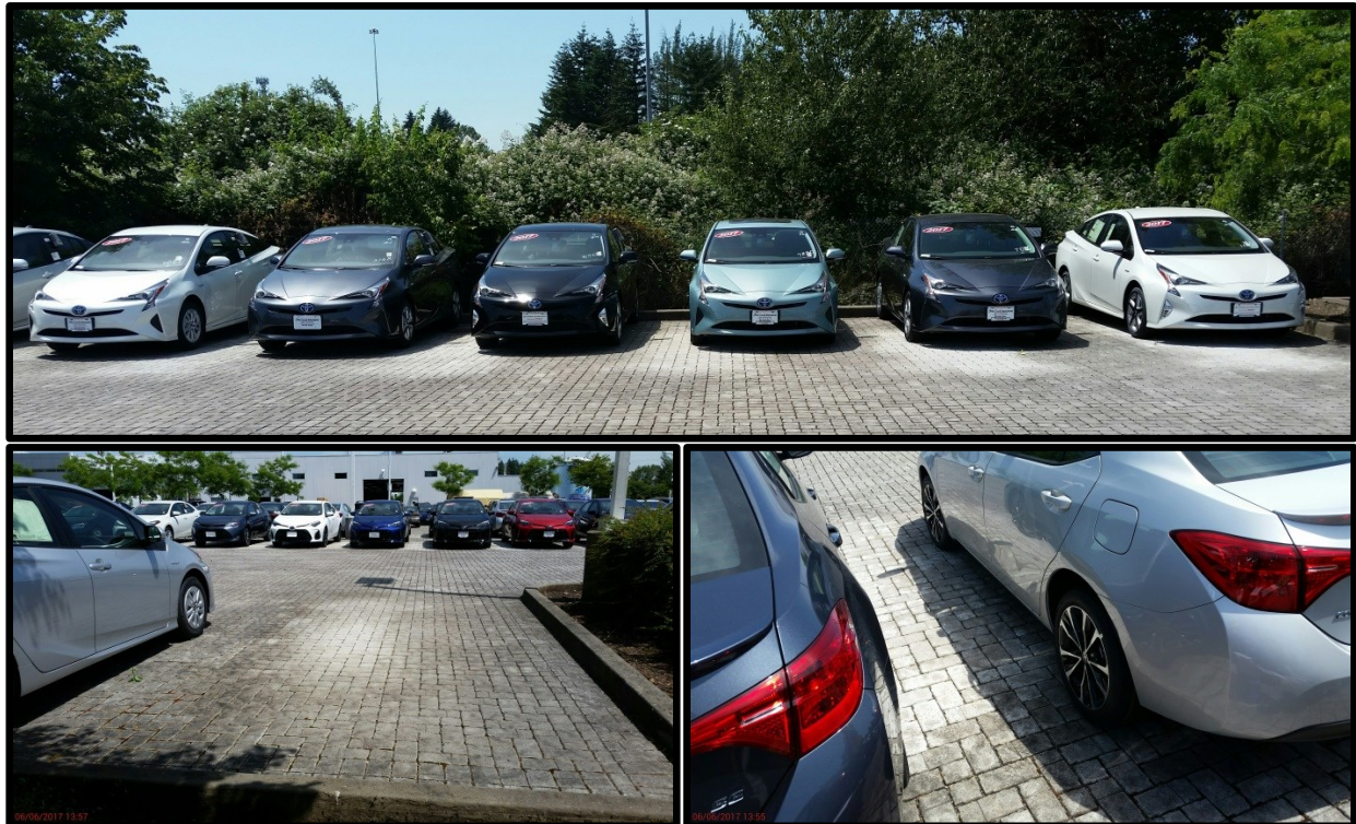
Figure 13. Examples of white appearance on pavers near new vehicles
