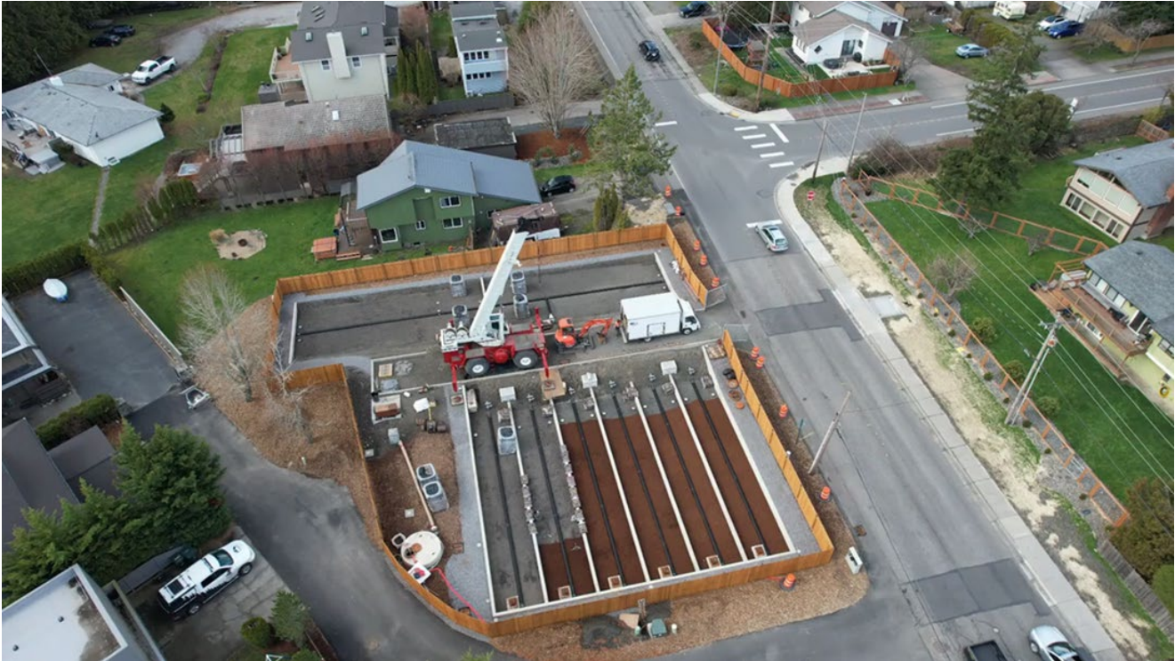
Figure 14. Construction of the Park Place Stormwater Phosphorus Treatment Facility, Bellingham, Washington.
