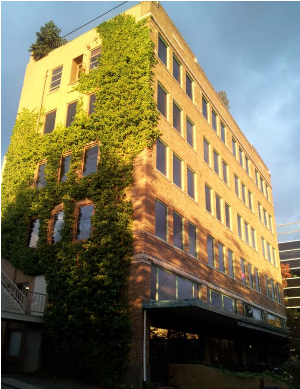
West and South facade
