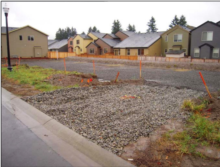
Figure 31: Small-scale Construction Entrance
