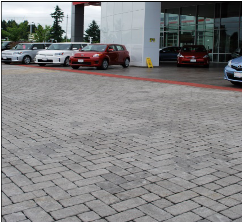
Figure 16: Permeable pavement application
