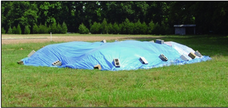
Figure 32: Covering a Stockpile
