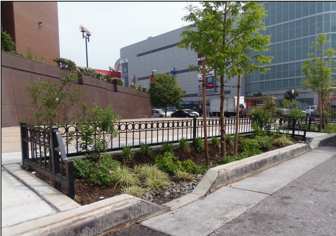
Figure 2.18: Example Pedestrian Rail System
