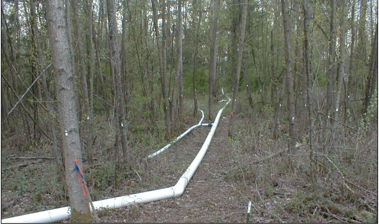
Figure 8.27: Manifold and Branches in a wooded, vegetated spray field
