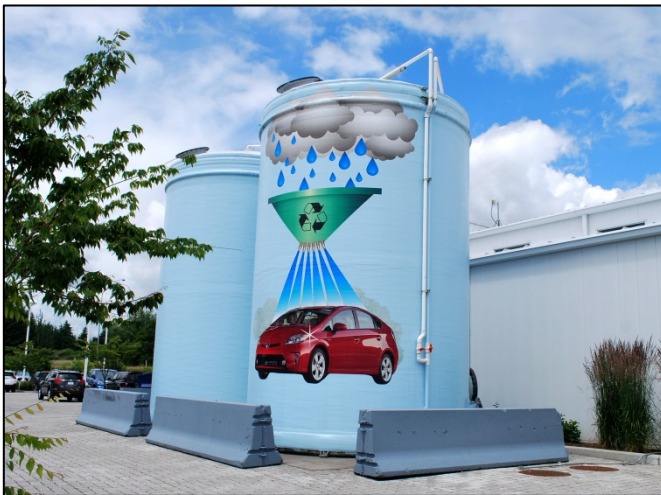
Figure 2.29: Cistern for Rainwater Harvesting
