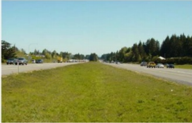
Figure 4.24: Compost-amended Vegetated Filter Strip Photo
