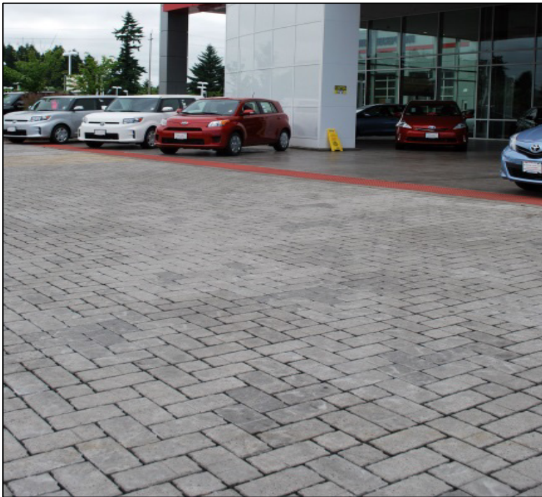
Figure 2.19: Permeable Pavement Application
