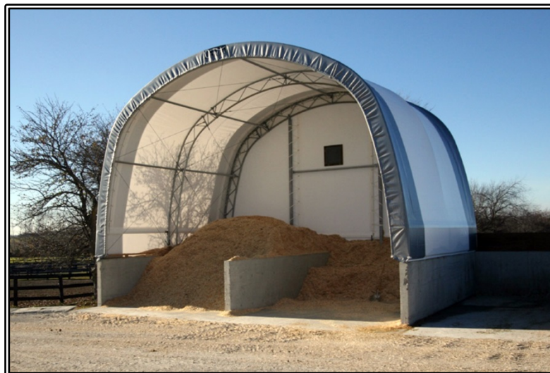
Figure 2.16: Covered Storage Area for Bulk Solids (include berm if needed)
