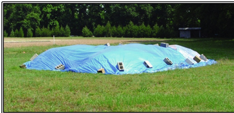
Figure 2.17: Material Covered with Plastic Sheeting
