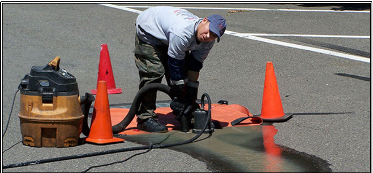
Figure 2.1: Collecting Washwater for Disposal
