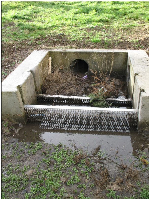
Sediment Trap with Accumulated Sediment
