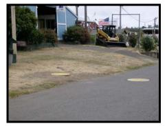
Ramp to Beef barn is too steep and inaccessible. A new ramp should be constructed from the entrance of the barn to the NE so that the slope of the pathway is no steeper than 1:12 and shall have a cross slope that does not exceed 1:48.
