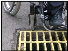
Wheelchair wheel can be easily inserted into the grate opening resulting in wheelchair falling over.
