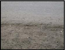
The pavement edge to the vendor displays on the south side of the horse riding arena are too high. Wheelchairs could easily fall over. Also, elevated edges are a potential trip and fall hazard.
