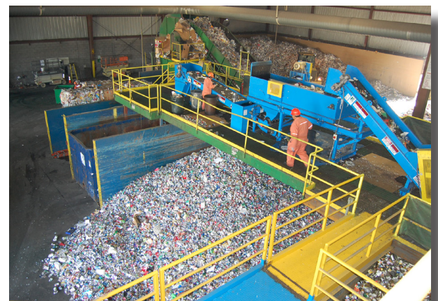
CRC Sorting Facility - Photo Source: City of Vancouver
