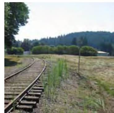
The eastern spur of the wye approaching Yacolt at MP-26.9.
