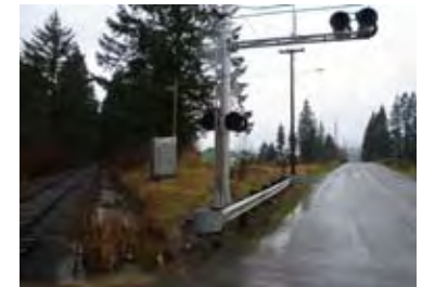
Most of the Chelatchie Rail crossings of roadways have warning signals similar to this one at NE 182nd Avenue.
