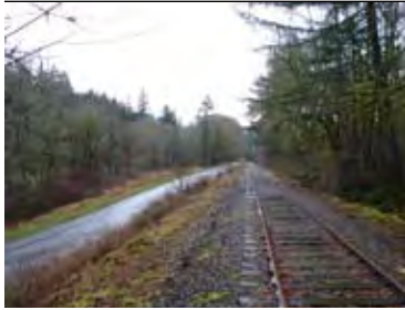
At MP-21.9, the corridor parallels NE Hantwick Road.
