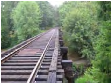
Trestle across Salmon Creek at MP-12.4.
