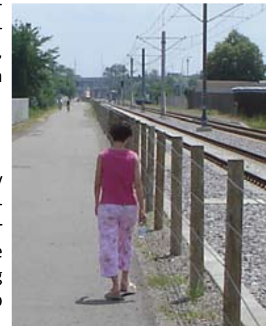
Simple wire fencing on a trail adjacent to high speed light rail. Hiawatha LRT Trail, Minneapolis, MN.
