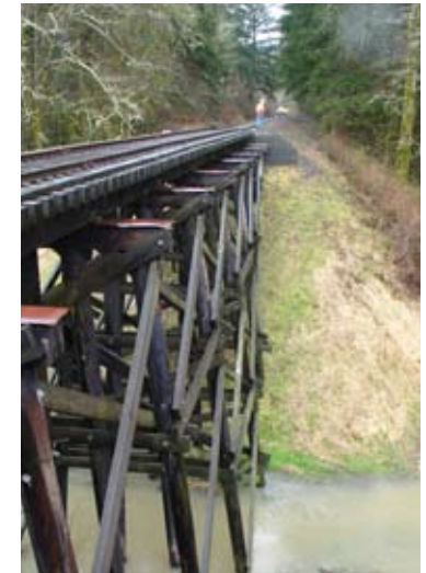
The design and condition of the existing Chelatchie Prairie Rail bridges make them unsuitable for the adding trail uses in combination with active rail operations. Bridge 18 south of Heisson.
