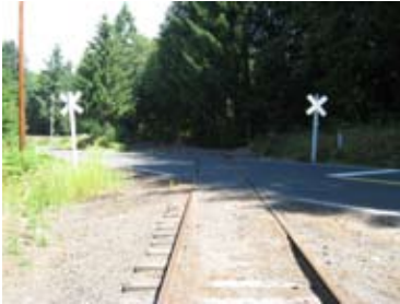
Crossing NE Amboy at MP 29.6.
