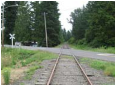
NE 259th crossing looking south.
