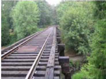
Trestle across Salmon Creek at MP-12.4.
