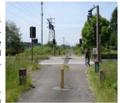
Properly located bollards approaching a Type II roadway crossing. Note the tall equestrian push button at right. Springwater Trail, Portland, OR.
