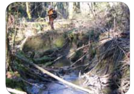
Urban streambank erosion
