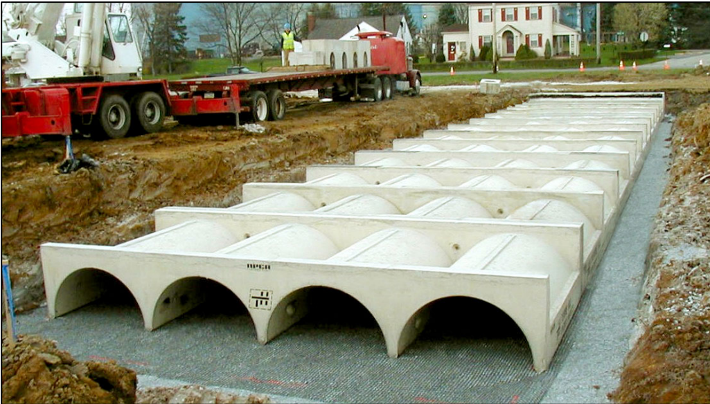
Example Proprietary Modular Detention System Installation
