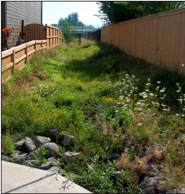
Example Typical Biofiltration Swale
