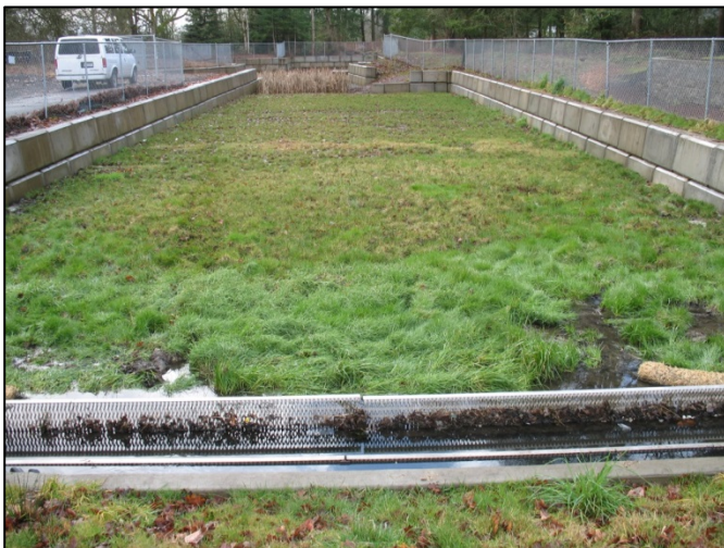
Example Typical Biofiltration Swale
