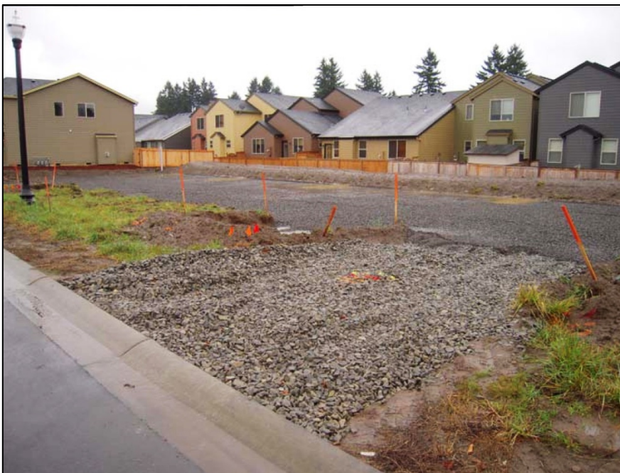
Figure 8.2: Small-scale Construction Entrance
