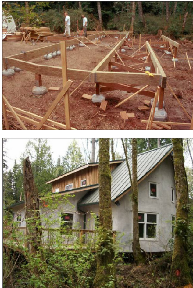
Figure 2.28: Pin Pier Foundation Construction & Completed Project, Bainbridge Island
