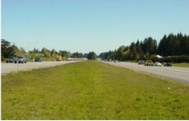
Figure 4.24: Compost-amended Vegetated Filter Strip Photo
