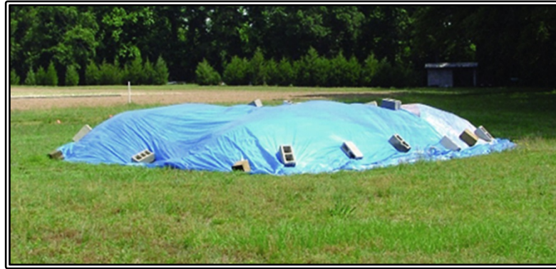
Figure 2.17: Material Covered with Plastic Sheeting
