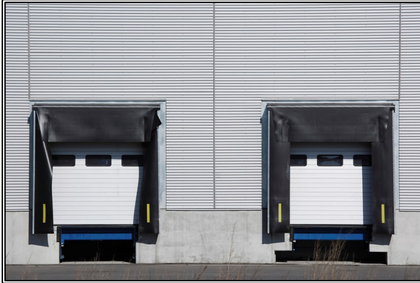
Figure 2.7: Loading Dock with Door Skirt
