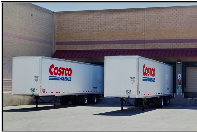
Figure 2.8: Loading Dock with Overhang
