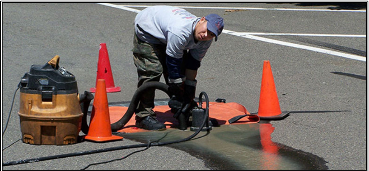
Figure 2.1: Collecting Washwater for Disposal
