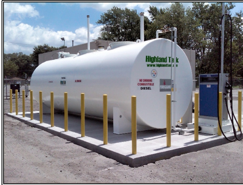
Figure 2.15: Above-ground Tank Storage
