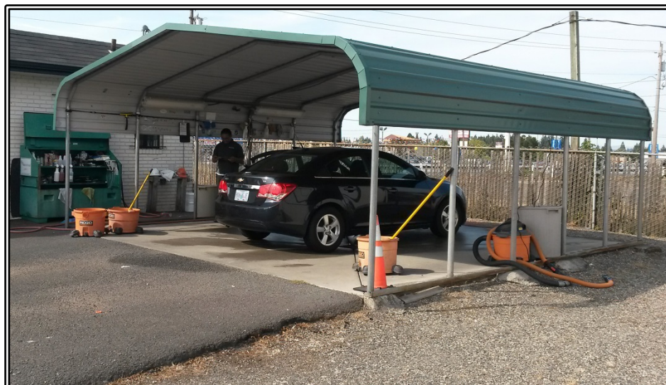
Figure 2.18: Covered Wash Area
