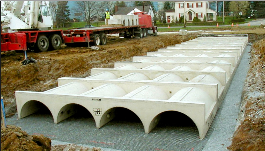
Example Proprietary Modular Detention System Installation
