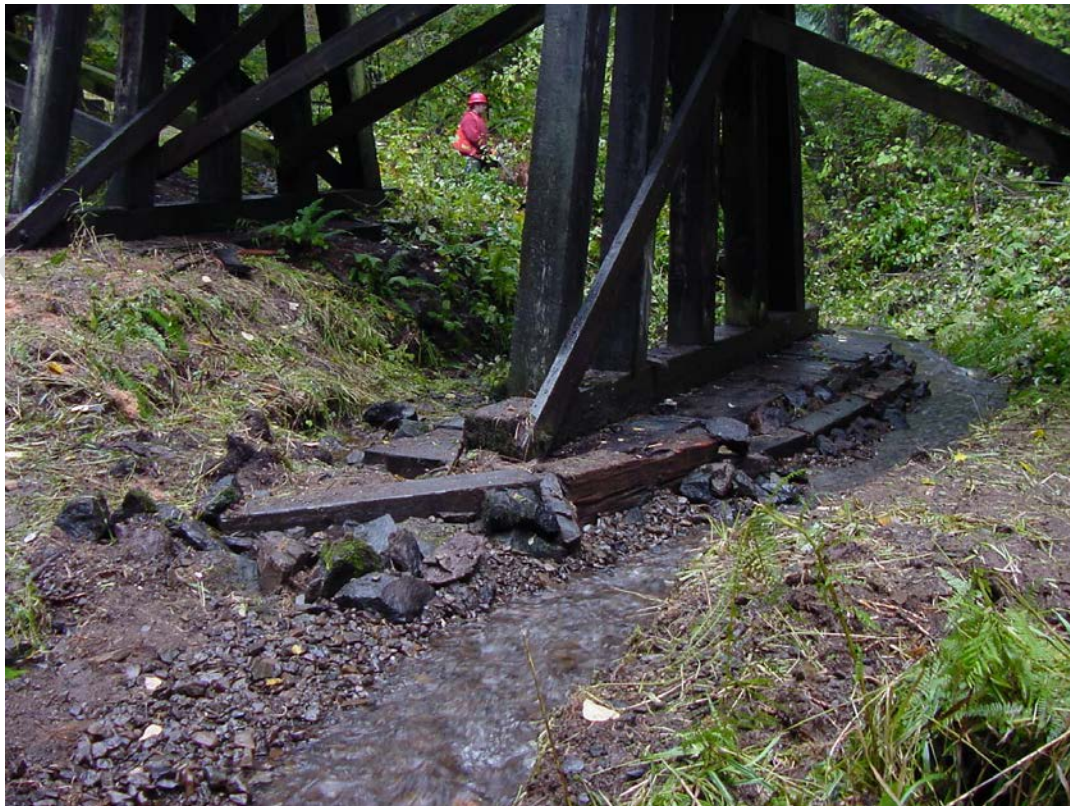
Figure 3 – View of Channel Looking Upstream Through Bridge
