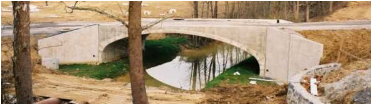
Figure 5, Example Arch Culvert Installation
