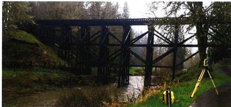
Figure 1, Existing Br. 12 Looking Upstream, Bent 1 to the right.
