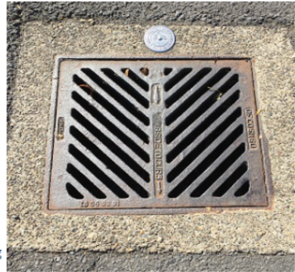
A catch basin, also known as a storm drain inlet, is designed to trap sediment and debris before it gets into the storm drainage system.
