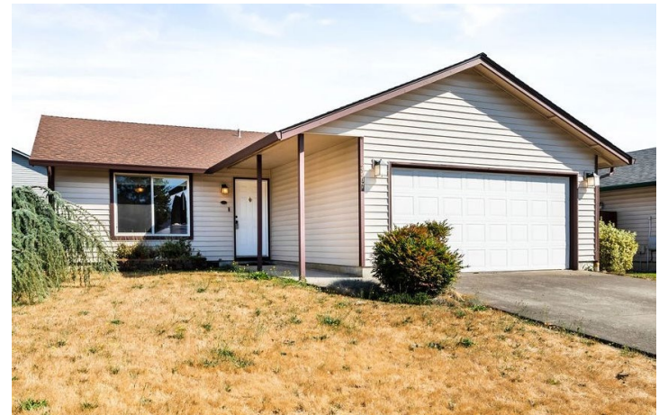
Proud Ground Community Land Trust model new home purchased 1 house = 4 low-income families achieve homeownership over the lifetime of the house.
