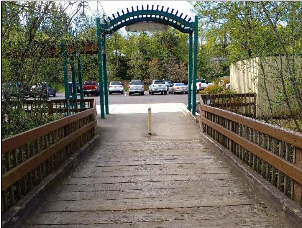
Figure 15. Overview of the project, area of previous ground disturbance at the bridge crossing Salmon Creek, view south.
