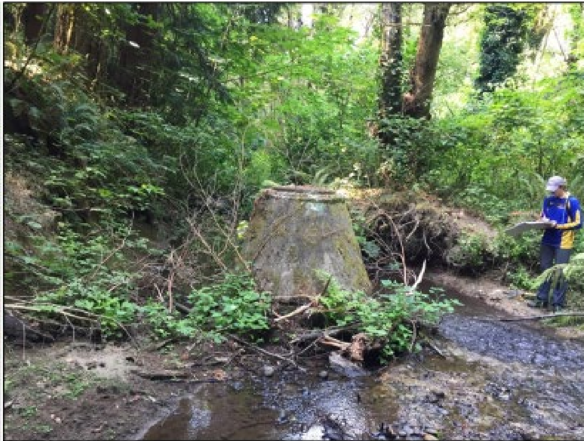
Exposed stormwater outlet within incised and straightened main channel (left) and an exposed manhole within the active channel of Cougar Creek (right) in the Cougar 3 project area.
