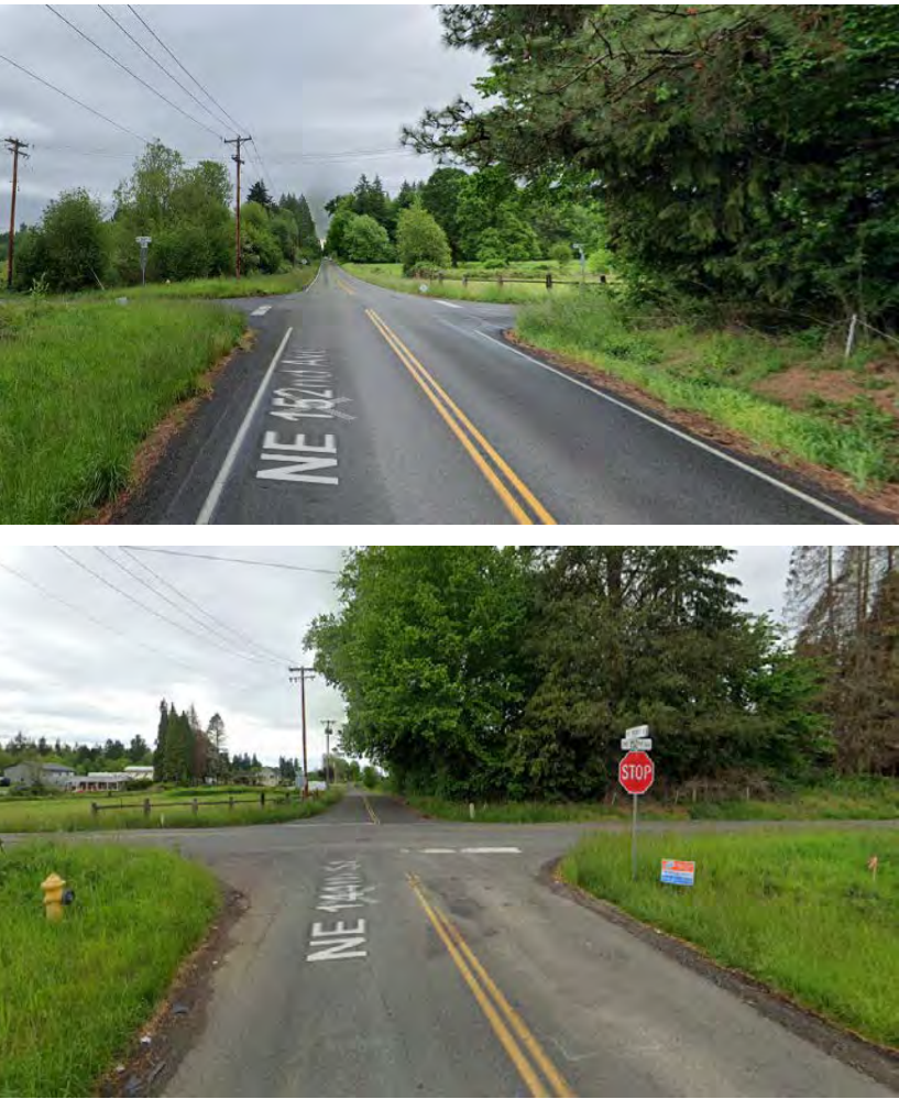
Photo I-1A Limited intersection sight distance due to vegetation
