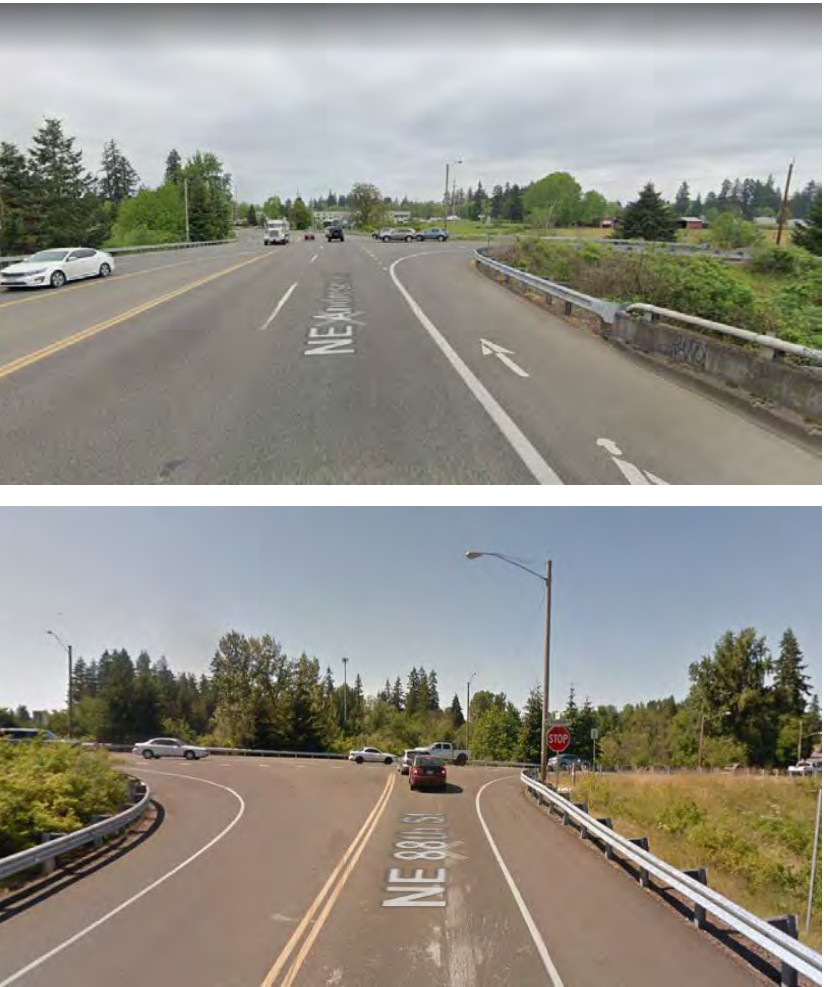
Photo I-1A: Minor approach on a crest curve Source: Google Earth, 2020.
