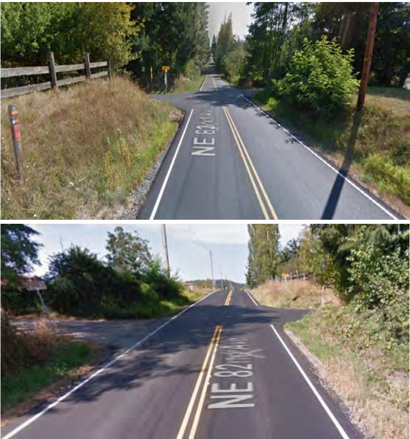
Photo I-1A Limited visibility due to sag curve Source: Google Earth, 2020.
