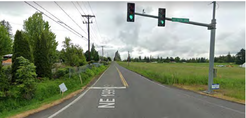
Photo I-1A Lack of left turn lanes on west and east legs of intersection
