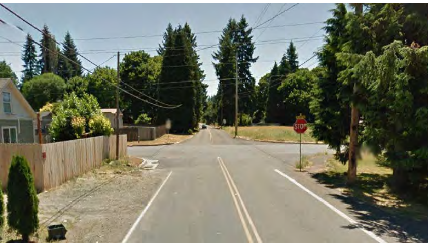
Photo I-IA Limited intersection sight distance because of Fencing Source: Google Earth, 2020.
