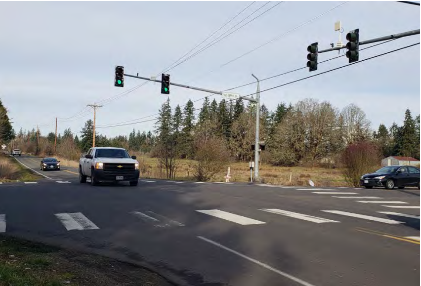
Photo I-IA: Lack of existing left turn lanes and tight turning radius
