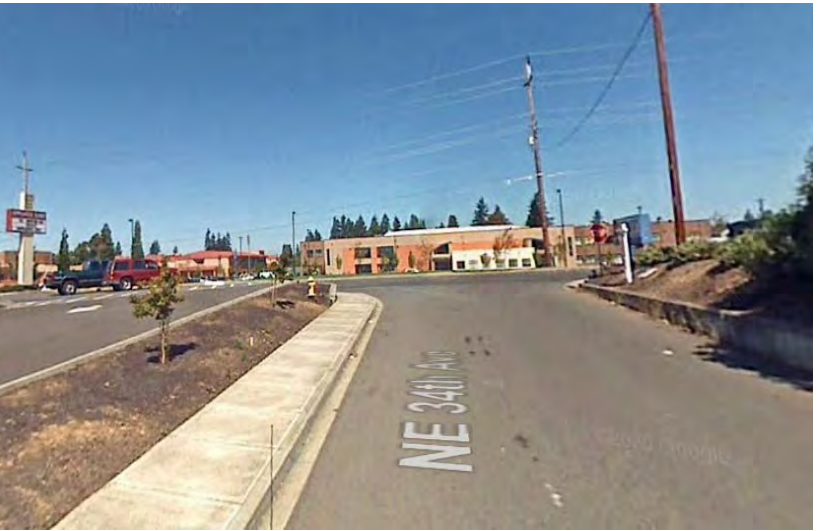
Photo I-IA Intersection on crest curve
