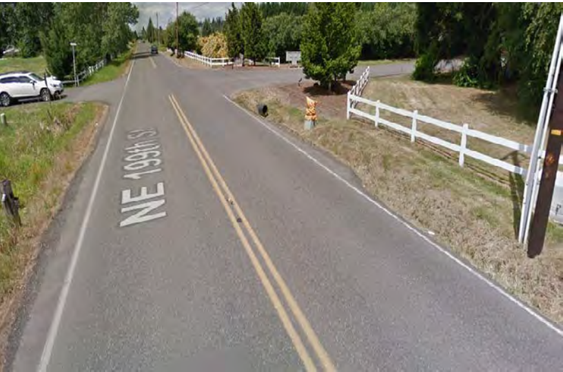
Photo I-IA: No definition of intersection approach on north leg
