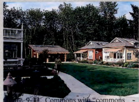
Figure 9-33. Commons with “commons room” shared by commons residents.
