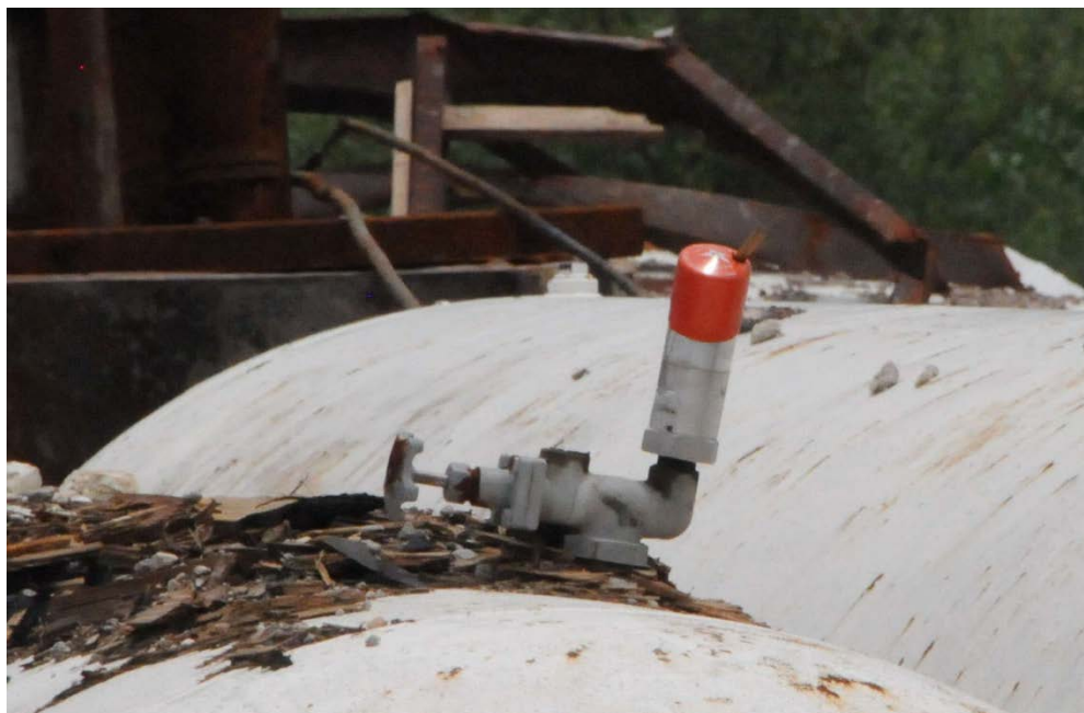
Figure 21. Anhydrous Ammonia Tank PRV, Post-Incident (Source: CSB)
