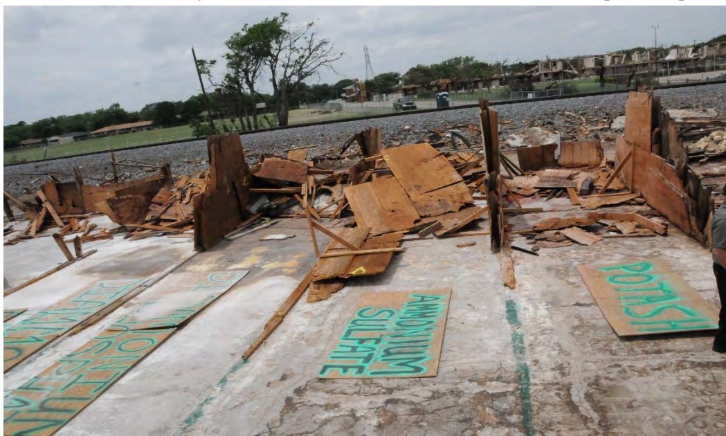
Figure 8. Plywood Bin Wall, Post-Explosion (Source: CSB)
