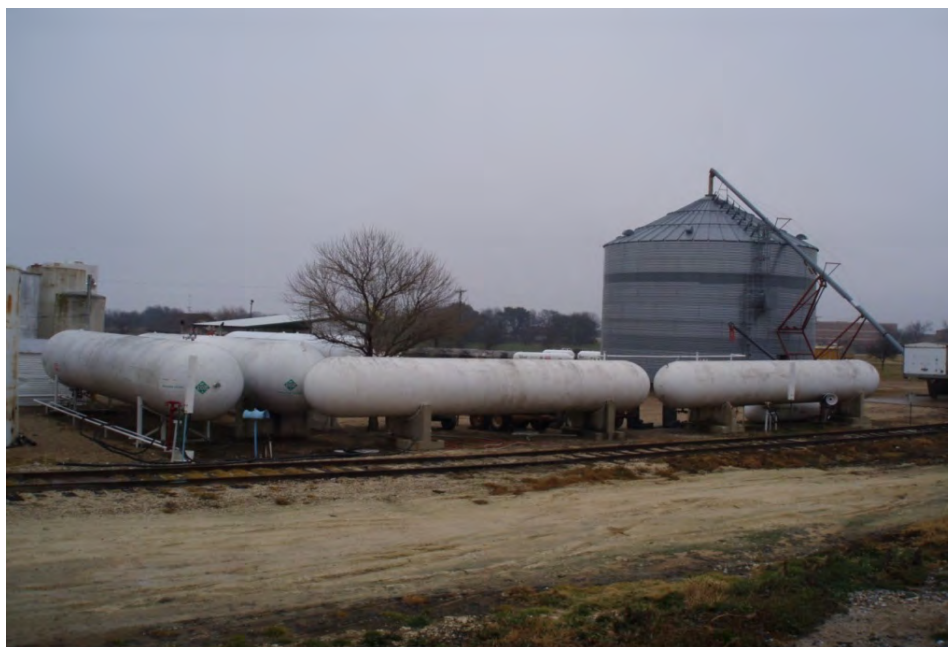
Figure 6. Anhydrous Ammonia Storage (Source: WFC Insurer)
