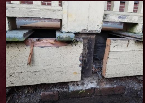
COLUMNS SIT ON DECKING AND ARE NOT INTERCONNECTED FLOOR-TO-FLOOR
