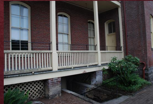
RETAINING WALL NEXT TO FOOTINGS WILL NEED TO BE REMOVED AND REPLACED.
