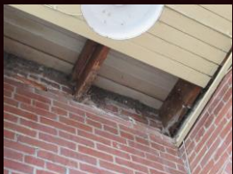
CONNECTION OF JOIST TO WALL IS DETERIORATED
