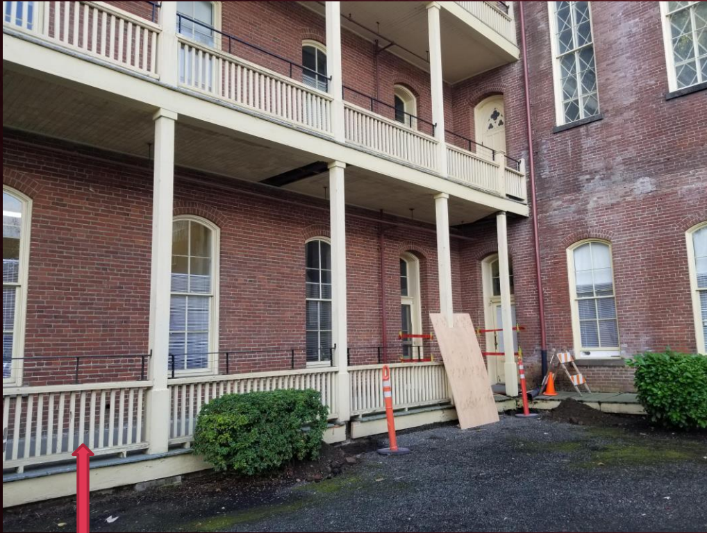
3-STORY PORCH SIMILAR TO WEST PORCH
