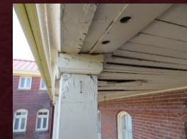
DETERIORATED SOFFITS
