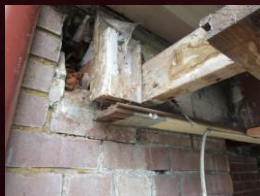
CONNECTION OF JOIST TO WALL IS DETERIORATED
