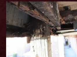
DETERIORATED SOFFITS
