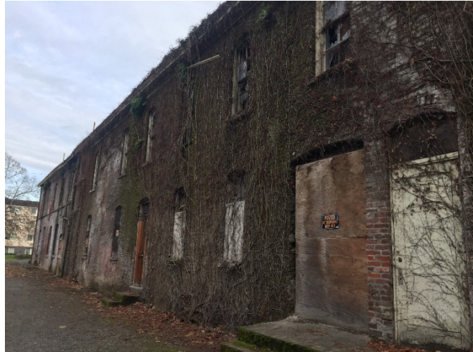
Laundry Building west elevation
