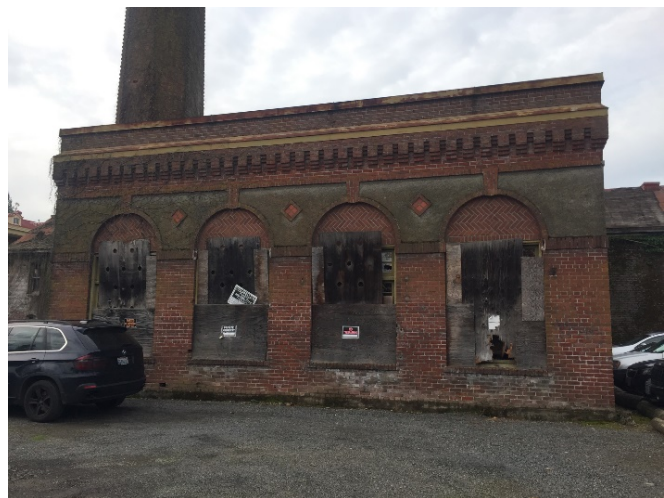
Boiler Building east elevation
