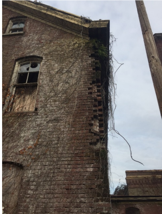
Laundry Building southeast corner detail of deteriorated brick
