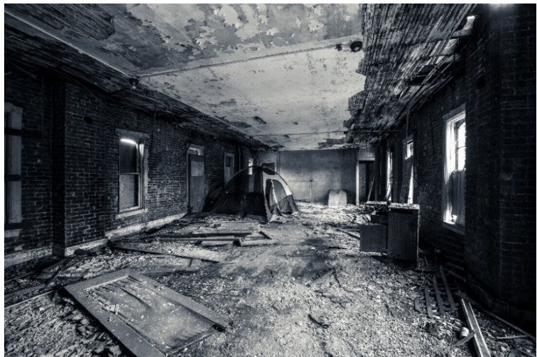
Laundry Building interior showing tent left behind by person experiencing homelessness
