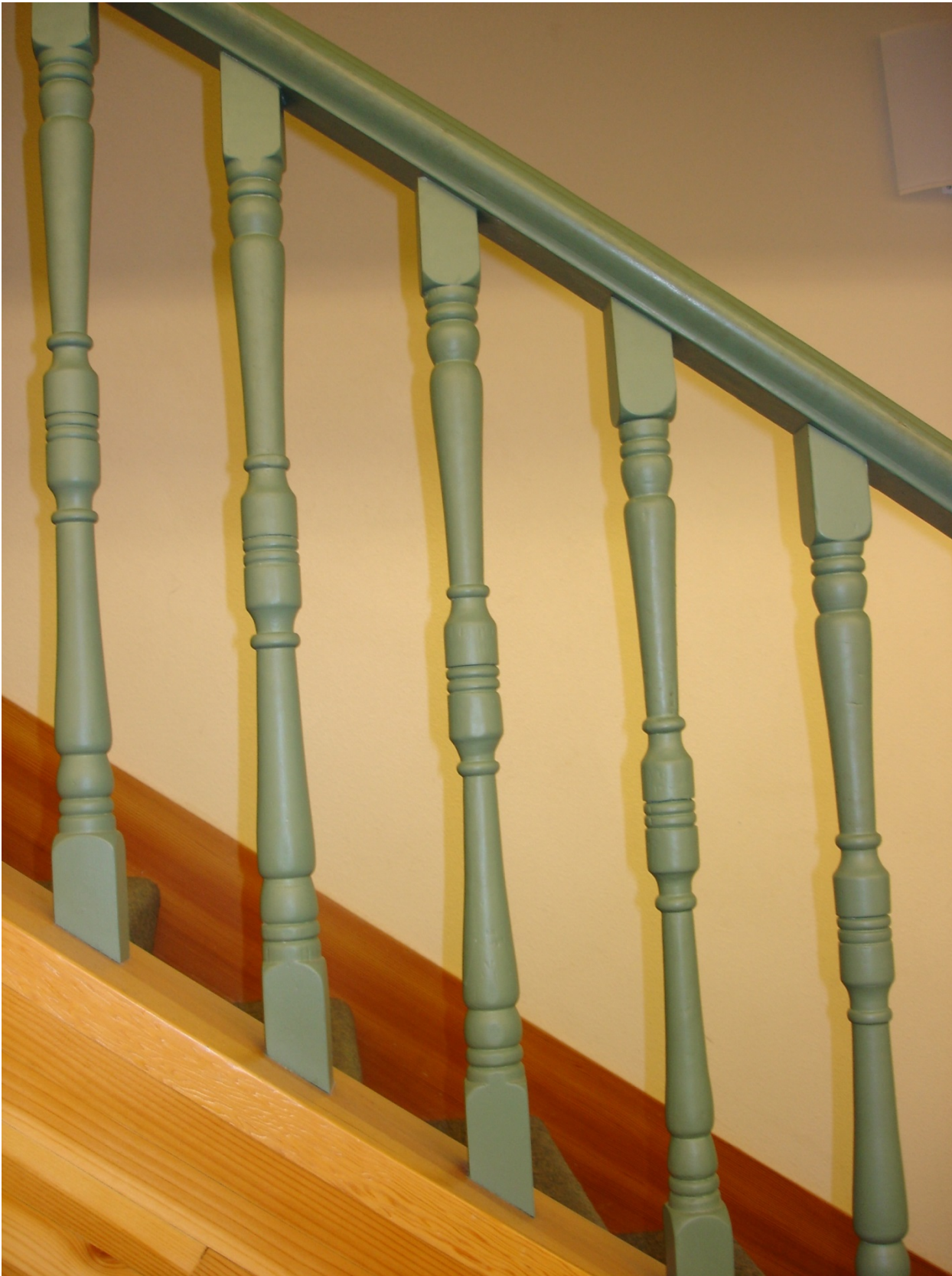
WA_Clark County_Zener House_21 Detail of central staircase balusters Date of photo: 6/16/2017 Photographer: Holly Chamberlain
