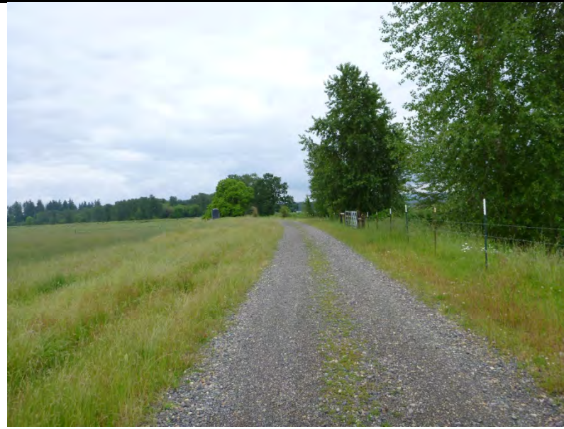
Photo point 3. Photo 2. From the crest of the Lewis River levee looking 275° down gravel access road.
