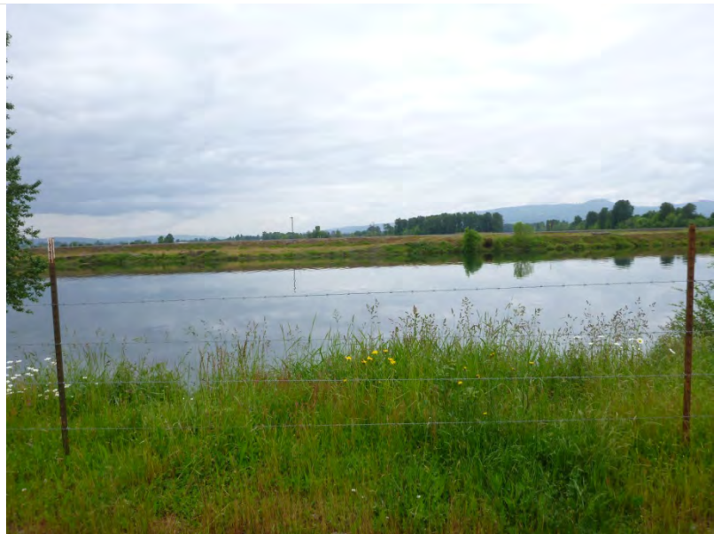
Photo point 3. Photo 2. From the crest of the Lewis River levee looking 340° at the Lewis River.
