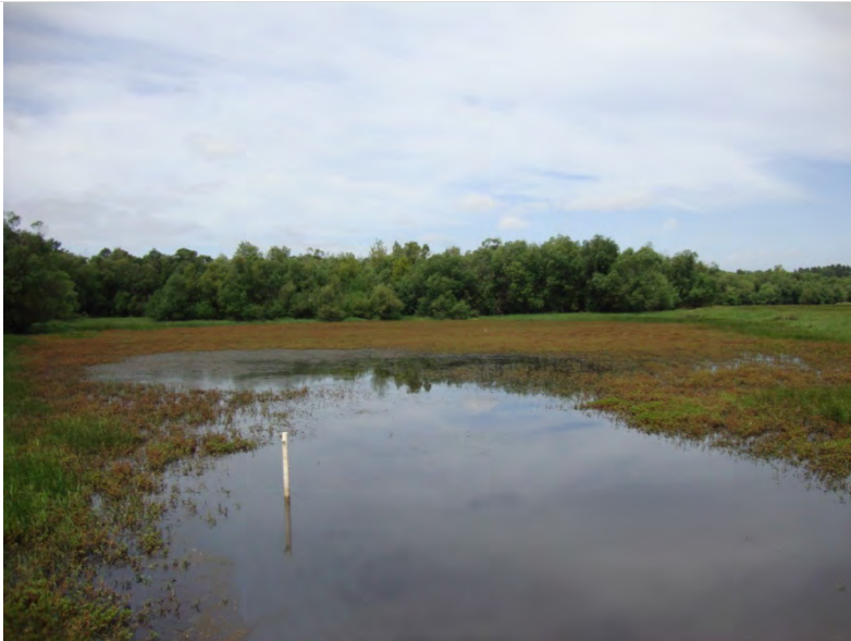
Photo point 35. Photo 1. From water control structure #1 at the west end of the rock-fill dam looking 340° at impounded water and water pepper and marsh seedbox wetland vegetation.
