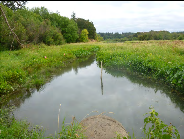
Photo point 43. Photo 1. From the southeastern end of the study site looking 120° at culvert outfall at the end of the waterfowl ponds draining into Gee Creek.
