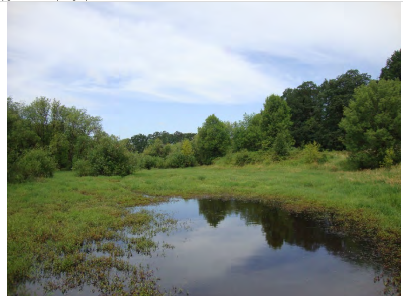
Photo point 37. Photo 1. From water control structure #2 at the east end of the rock-fill dam looking 340° at impounded water and water pepper and marsh seedbox wetland vegetation.
