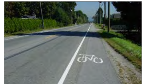
Figure 6. Shoulder bikeways accommodate cycling on rural roads without curbs and gutters.
