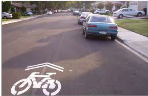
Figure 8. Shared lane markings are used to indicate a bicycle route, and to show cyclists where they should be riding in the road.
