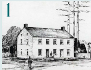
1 Clark County's first courthouse was a two-story, wood frame structure built in 1855 on West Reserve Street, near Fort Vancouver. Cost: $1,000 CCHM Collection 01006
