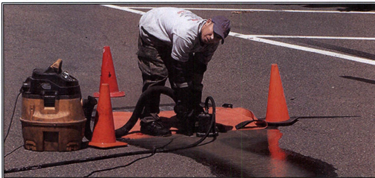
Figure 2.1: Collecting Washwater for Disposal
