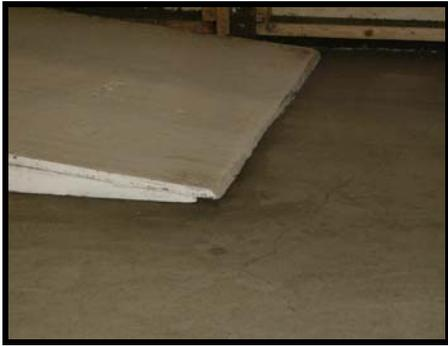
Ramp on west end of horse riding arena to elevated spectator platform appears to be too steep. The edge of the ramp on the floor is too high – Approx 1" lip.
