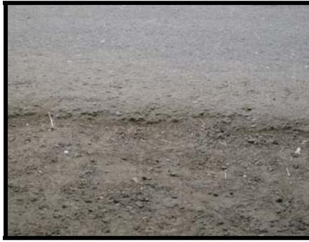
The pavement edge to the vendor displays on the south side of the horse riding arena are too high. Wheelchairs could easily fall over. Also, elevated edges are a potential trip and fall hazard.
