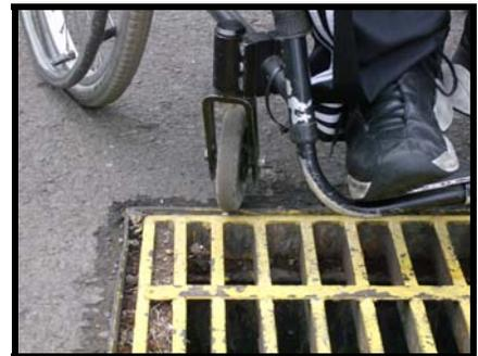
Wheelchair wheel can be easily inserted into the grate opening resulting in wheelchair falling over.
