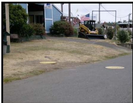
Ramp to Beef barn is too steep and inaccessible. A new ramp should be constructed from the entrance of the barn to the NE so that the slope of the pathway is no steeper than 1:12 and shall have a cross slope that does not exceed 1:48.
