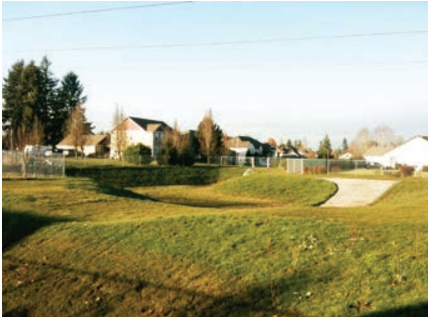
2008-2012 Stormwater CIP: Grassland Meadows Stormwater Facility Retrofit
