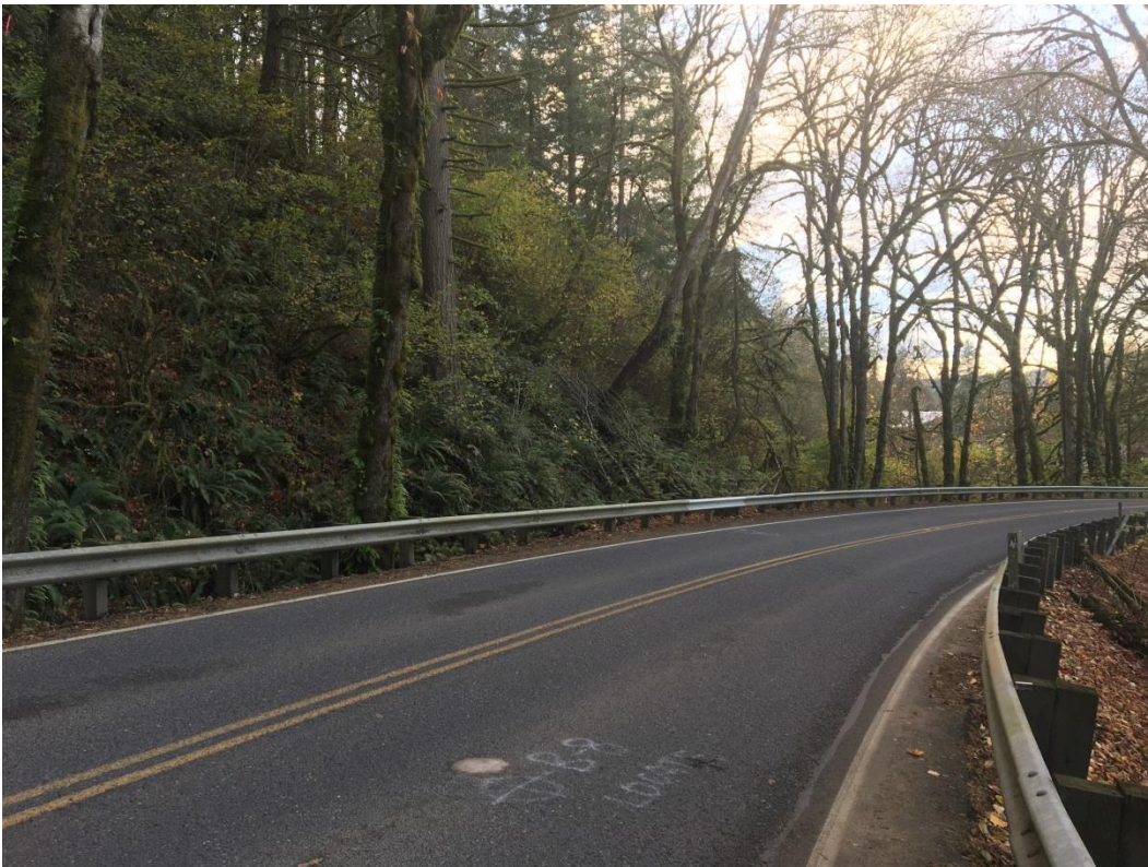
Steep Bank at West Side of Roadway
