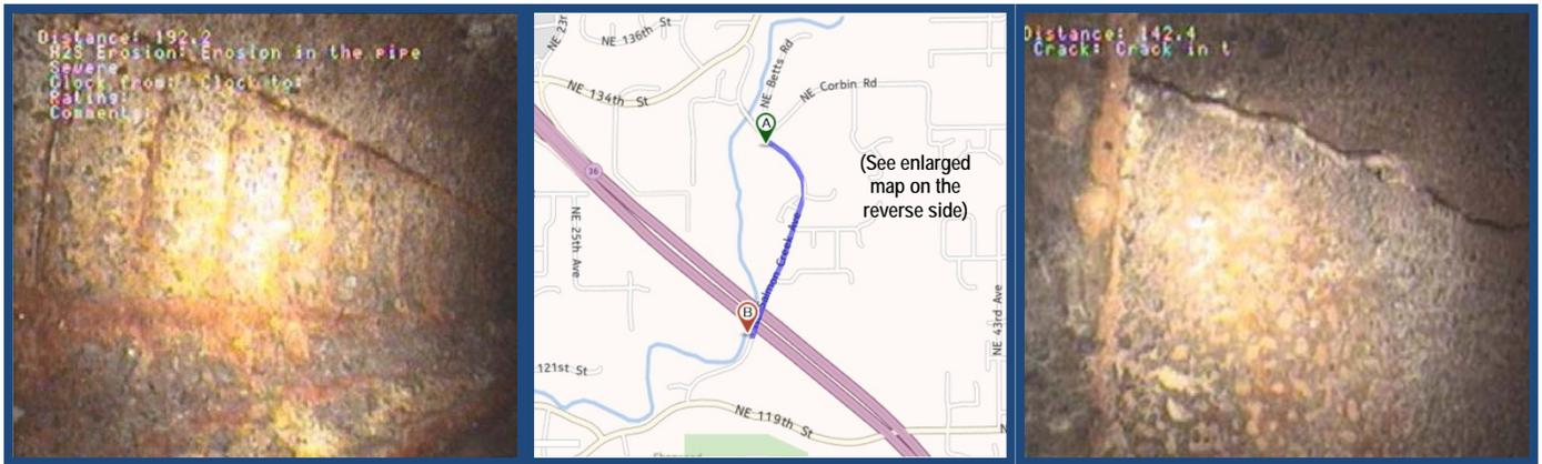
*Erosion in the Pipe – Near Corbin Road*
