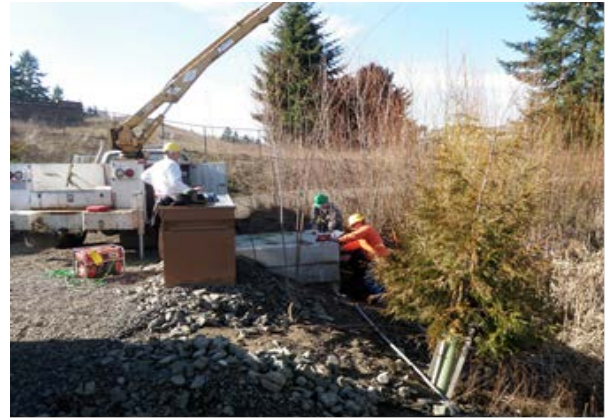
Crews install weir at a treatment wetland BMP monitoring site
