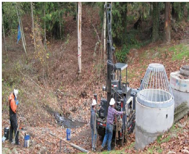
Encore Stormwater Facility Retrofit
