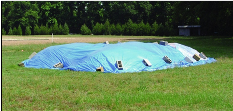
Figure 30: Covering a Stockpile
