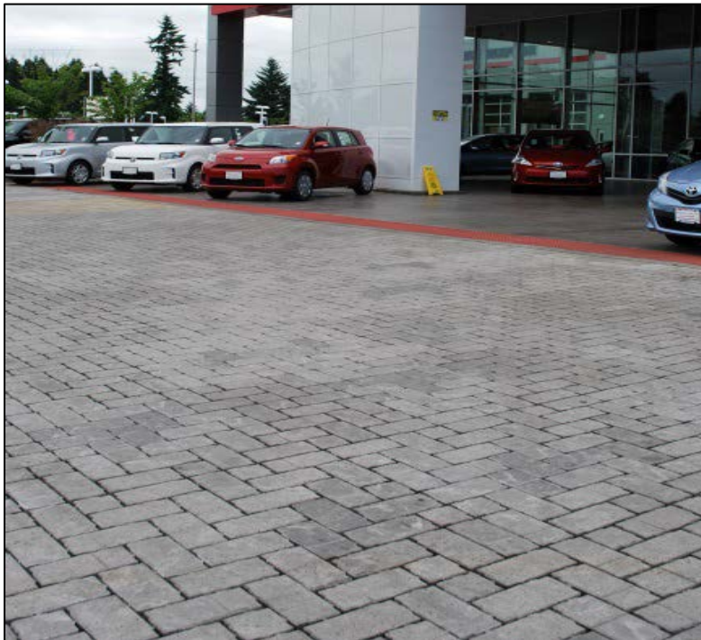
Figure 14: Permeable pavement application
