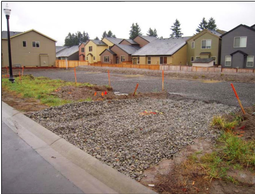
Figure 29: Small-scale Construction Entrance
