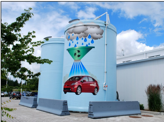
Figure 2.28: Cistern for Rainwater Harvesting
