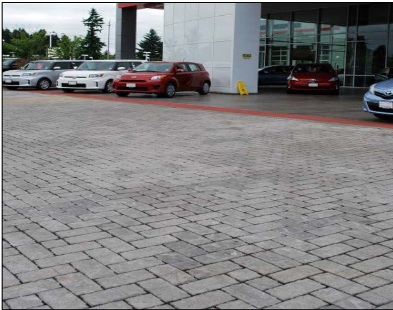
Figure 2.18: Permeable Pavement Application
