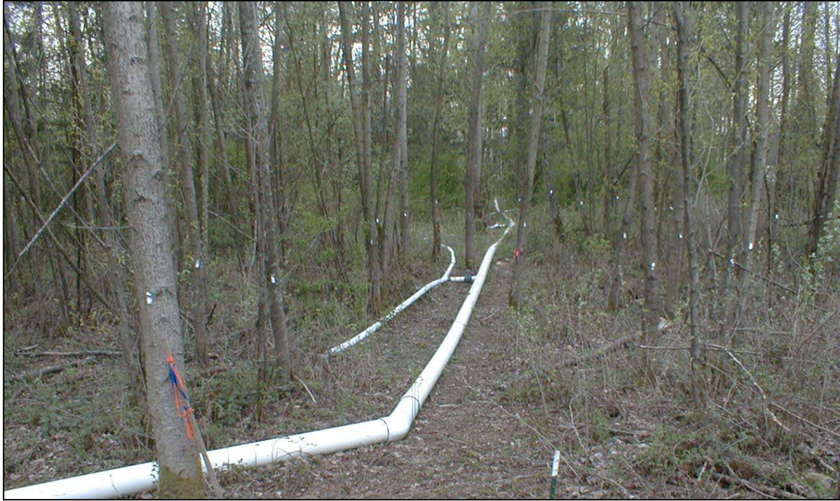
Figure 9.27: Manifold and Branches in a wooded, vegetated spray field (Source: SMMWW)
