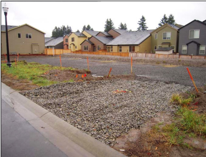
Figure 9.2: Small-scale Construction Entrance
