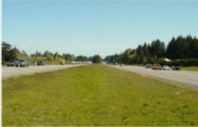
Figure 4.24: Compost-amended Vegetated Filter Strip Photo
