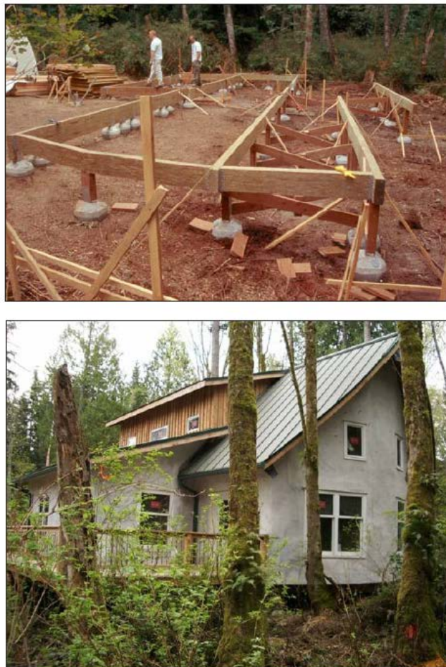
Figure 2.27: Pin Pier Foundation Construction & Completed Project, Bainbridge Island
