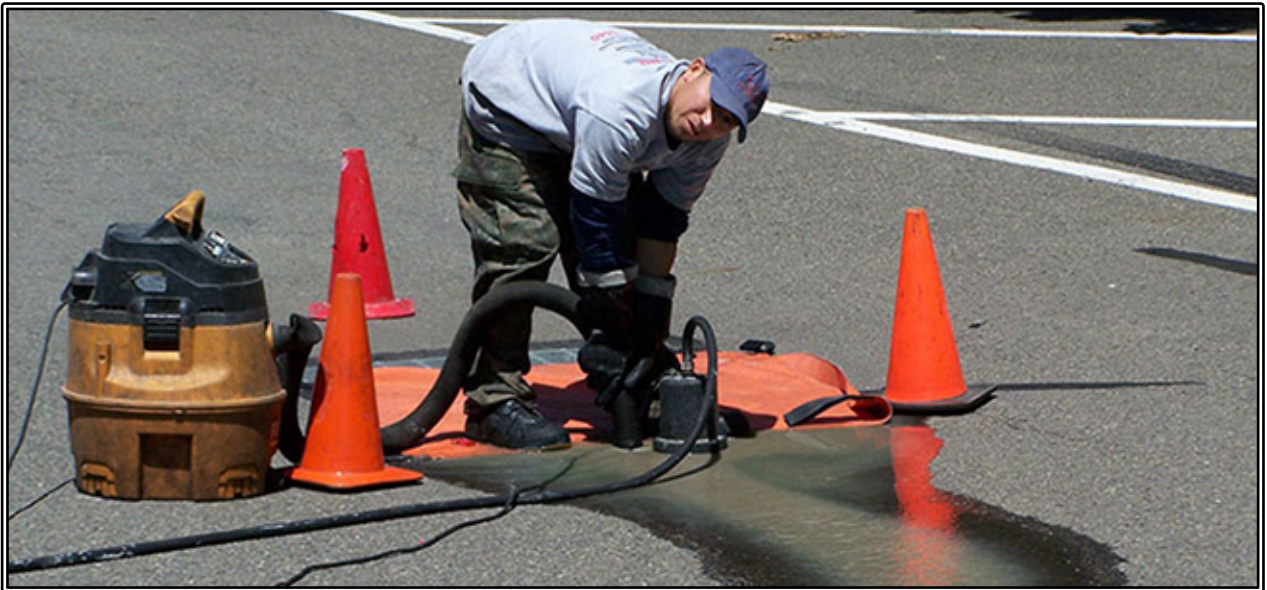
Figure 2.1: Collecting Washwater for Disposal
