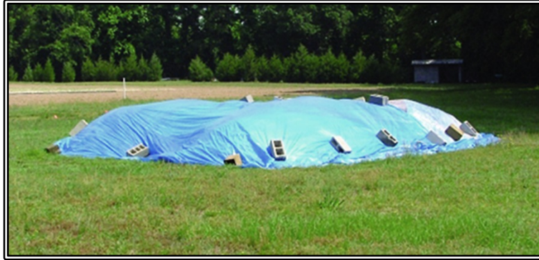
Figure 2.17: Material Covered with Plastic Sheeting
