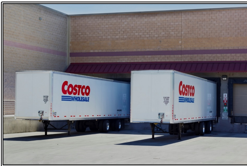
Figure 2.8: Loading Dock with Overhang
