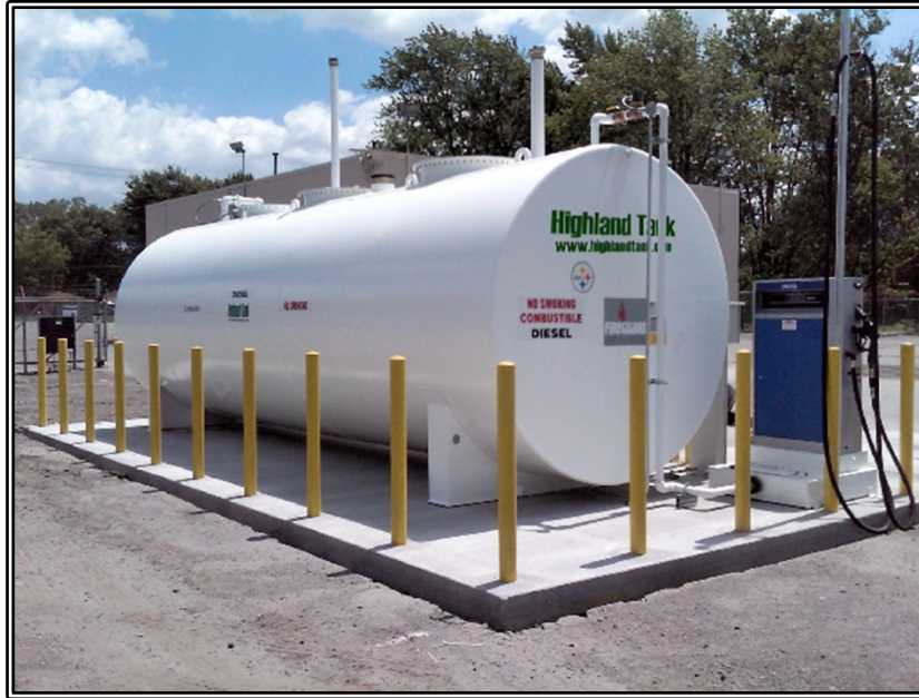
Figure 2.15: Above-ground Tank Storage
