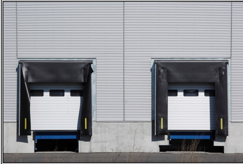
Figure 2.7: Loading Dock with Door Skirt
