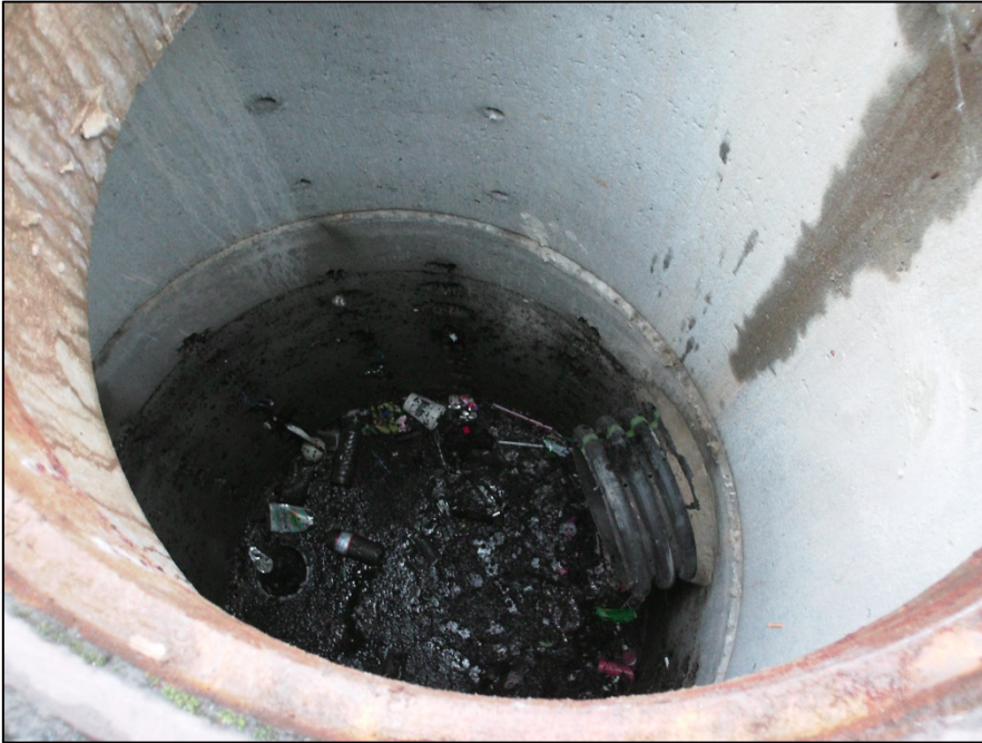
Drywell with Accumulated Trash
