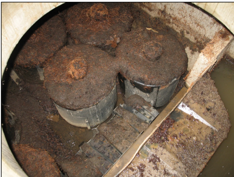
Media Cartridge Filter Vault with Accumulated Sediment
