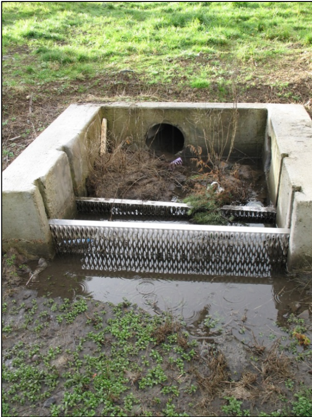
Sediment Trap with Accumulated Sediment
